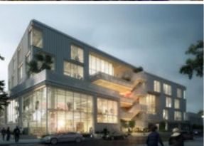
717 SEWARD ST 83K SF | UNDER CONSTRUCTION
