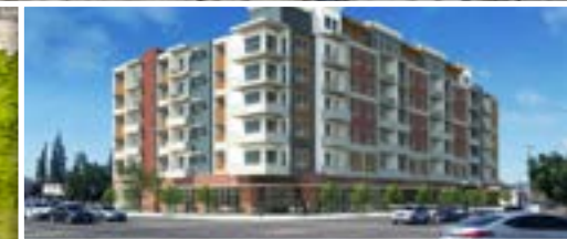
6801 CANOGA AVE 203 UNITS | UNDER CONSTRUCTION 3.95 FAR | 8 STORIES
