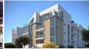
CHESTNUT APARTMENTS 24 UNITS | UNDER CONSTRUCTION
