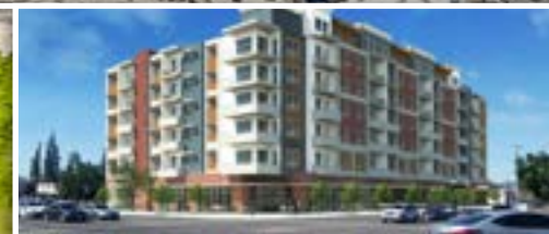
6801 CANOGA AVE 203 UNITS | UNDER CONSTRUCTION 3.95 FAR | 8 STORIES
