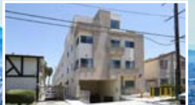
6816 INDEPENDENCE AVE 18 UNITS | BUILT IN 2016 3 STORIES
